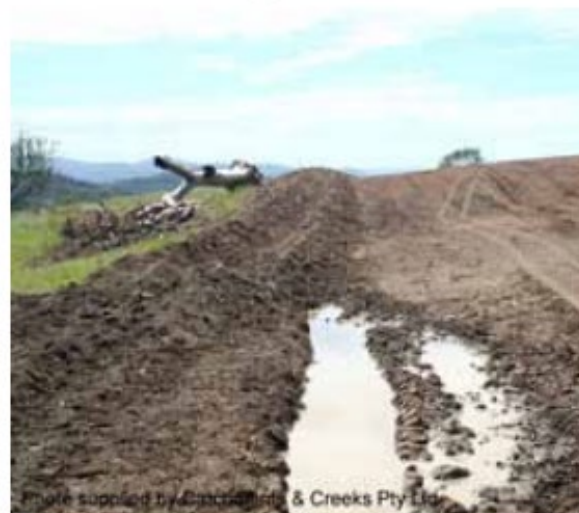
Flow diversion bank
