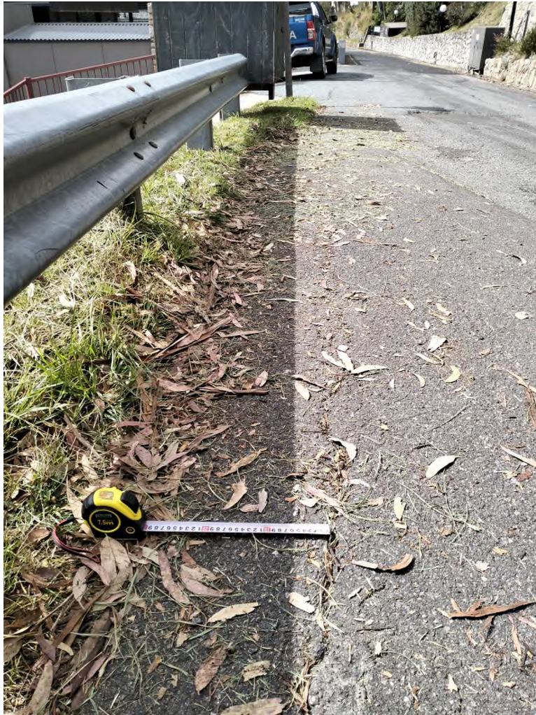
KOSCIUSZKO THREDBO PTY LTD PROPOSED DEMOLITION & REDEVELOPMENT - SONNBLICK LODGE – 10 BOBUCK LANE, THREDBO, NSW SITE PHOTOGRAPHS – TENSION CRACKS ON THE ROAD PAVEMENT
