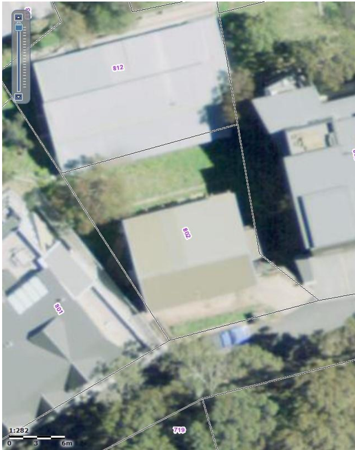
KOSCIUSZKO THREDBO PTY LTD PROPOSED DEMOLITION & REDEVELOPMENT - SONNBLICK LODGE – 10 BOBUCK LANE, THREDBO, NSW RECENT AERIAL PHOTOGRAPH
